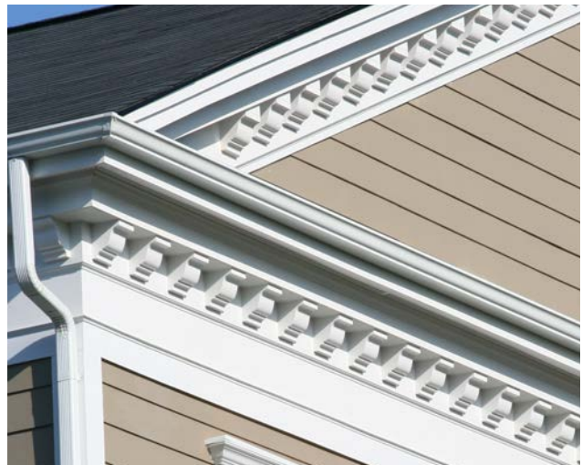
Figure 920-55: Cornice with Dentils
