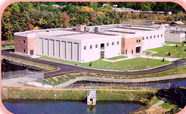
Millwood Water Treatment Plant: Example of Governmental Energy Consumption in New Castle
