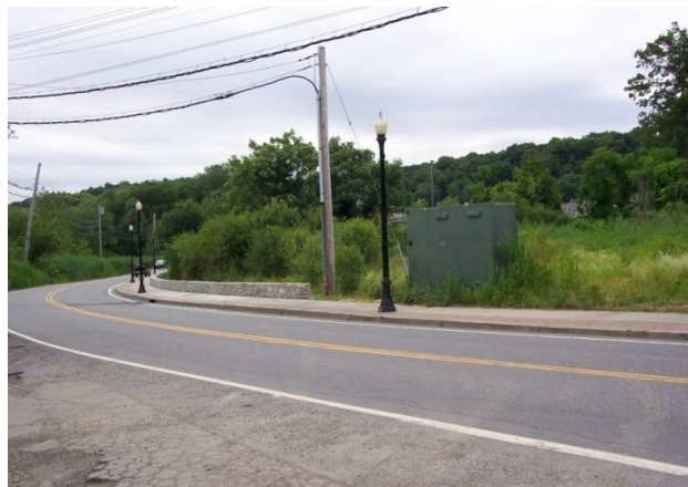
Finished sidewalk and stone wall on Station Place
